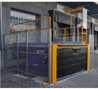
Truck dock with motor powered roller deck for 10ft ULD's.
